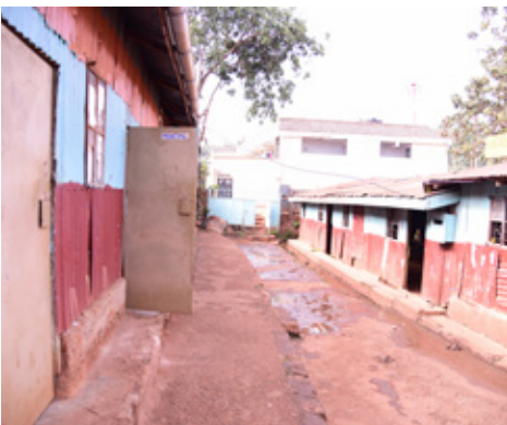
The Principal's Office is seen, tucked in a row of other corrugated iron structures within the school compound.
